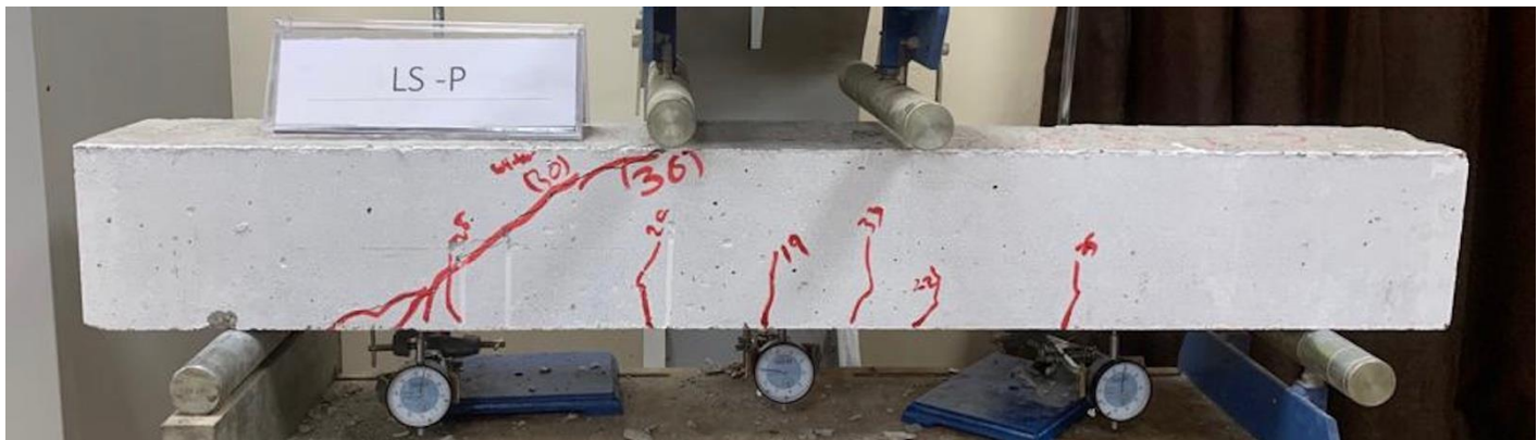
Fig. 10 Crack pattern at failure of beam LS-P.
