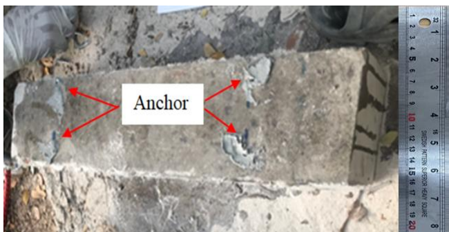
Fig. 3: Beam strengthened with LoC-GFRP with additional support from epoxy-based anchors.
