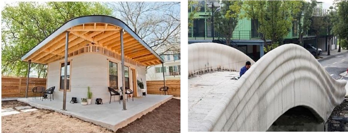
Fig. 15 (a) In-situ house and (b) Prefab bridge constructed using 3D-printed concrete. Reproduced with the permission from [148], Copyright 2020 The Authors.
