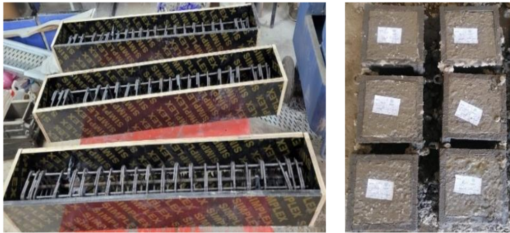
Fig. 4 Casting of beams and cubes.
