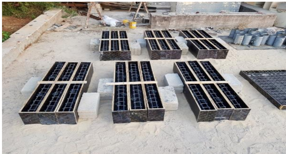
Fig. 3 Casting molds fastened and prepared for concrete casting on a sand surface.
