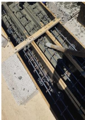
Electric concrete vibrator
