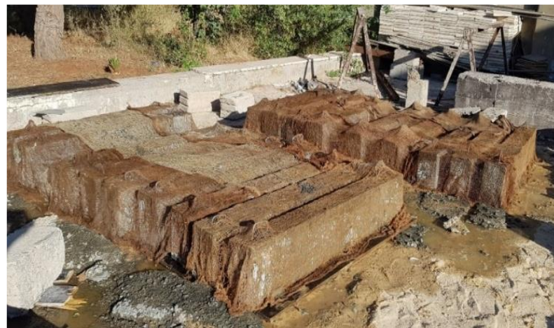
Beams covered in burlap for curing
