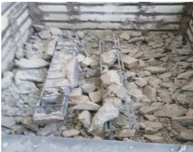
Fig. 18 Explosive spalling of beam specimens.
