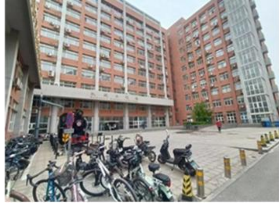
(b) Actual front view of the Mechanical Building.
