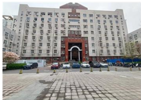
(d) Actual front view of the Civil Engineering Building.
