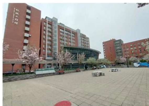
(f) Actual rear view of the Mechanical Building.
