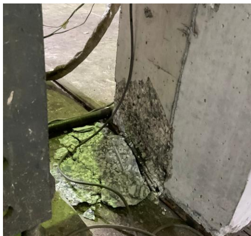
Fig. S3: Concrete crushing observed in Specimen ES-20.
