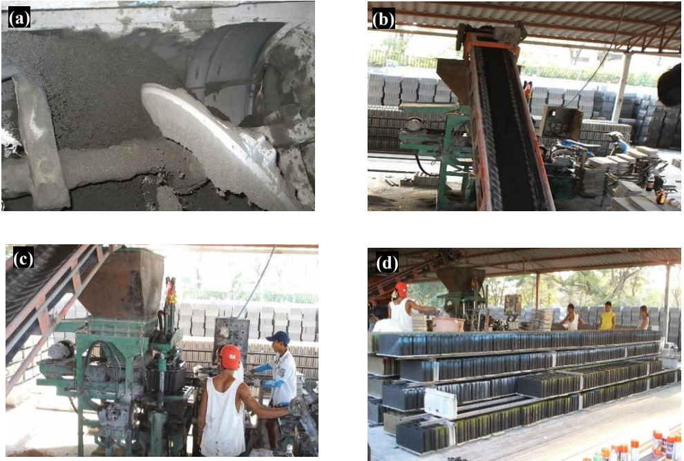
Fig. S2: Hollow concrete blocks manufacturing process: (a) mixing, (b) conveying, (c) vibrating press, and (d) drying.
